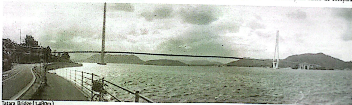
Tatara Bridge (1.480m.)
